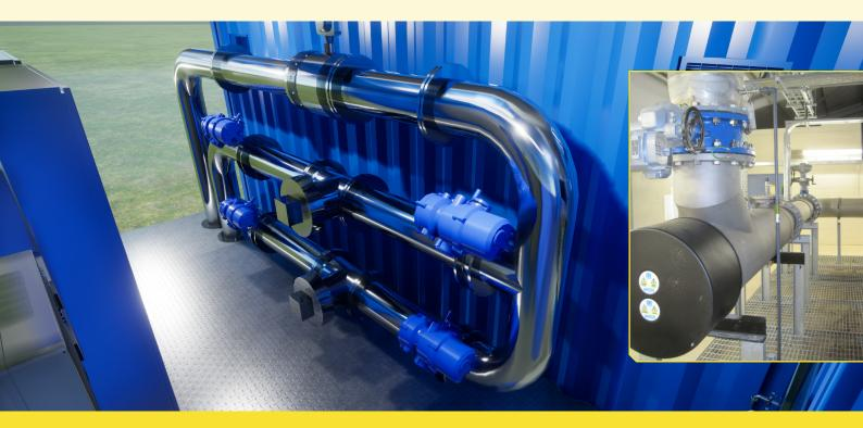
Each 20ft container can utilise various bespoke layouts to accommodate existing, external, site pipework arrangements, providing clear access to all areas. For new site installations, a standard floor entry/exit pipework arrangement would be incorporated for a more secure system.
